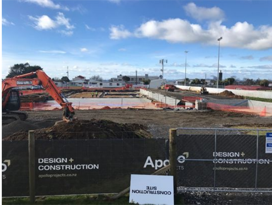
Figure 10: Slab completion and blockwork underway
