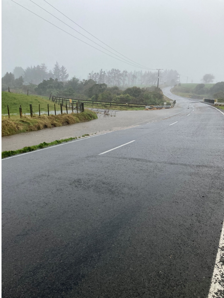
Figure 1: Flooding on Opunake Road.
