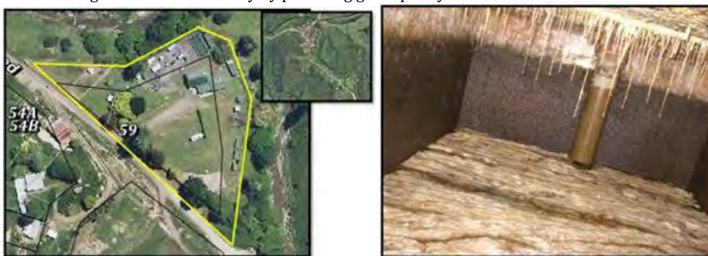
Figure 30 - Whangamomona Septic Tank and Fat Build Up
