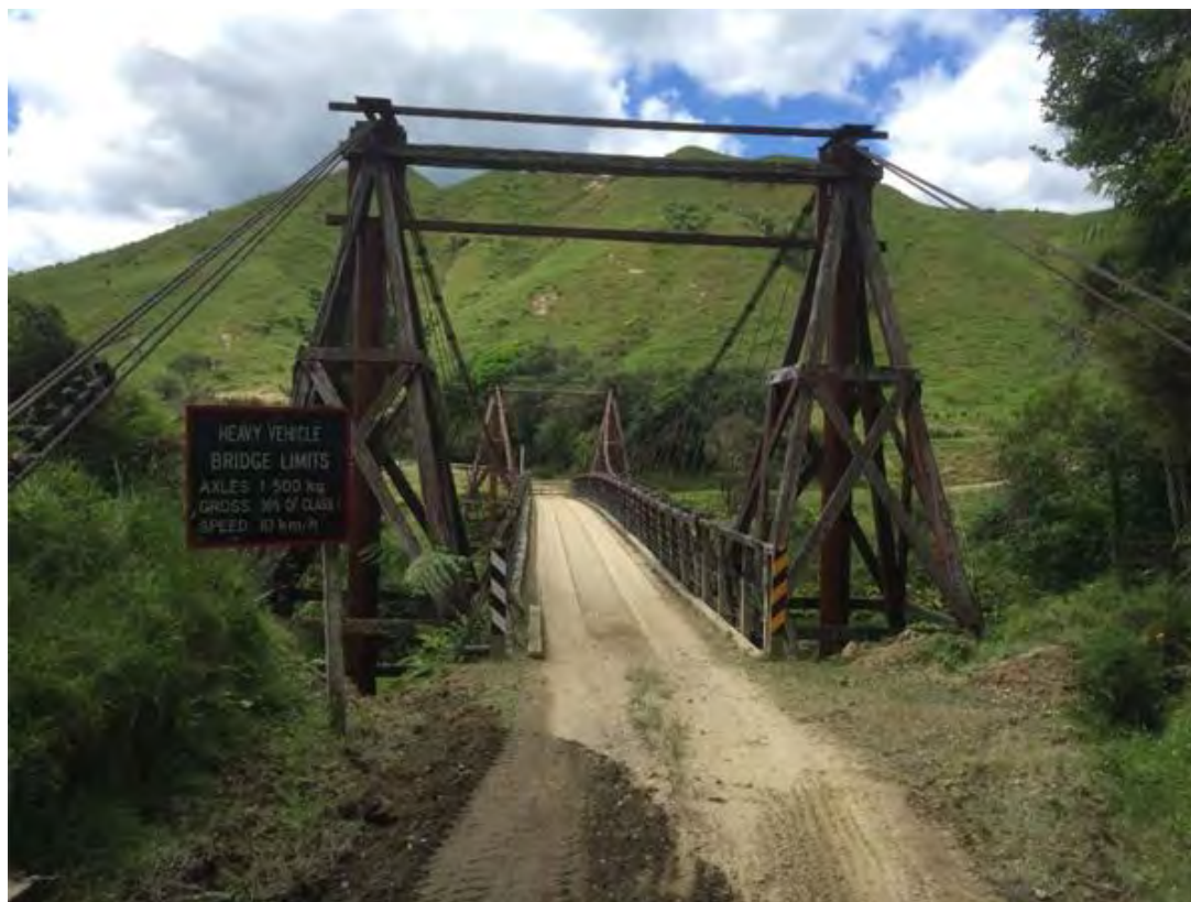
Figure 38 - Lower Kohuratahi Road Bridge
