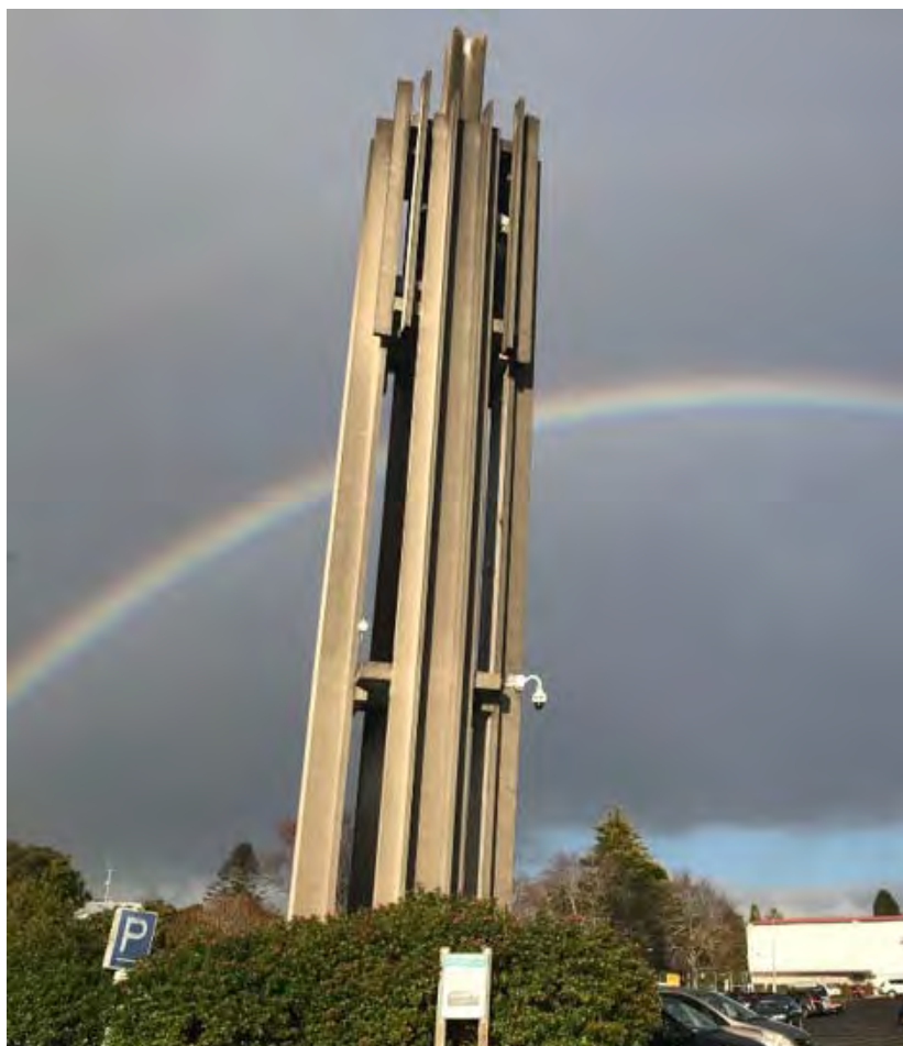
Figure 34 - Bell Tower, Miranda Street, Stratford
