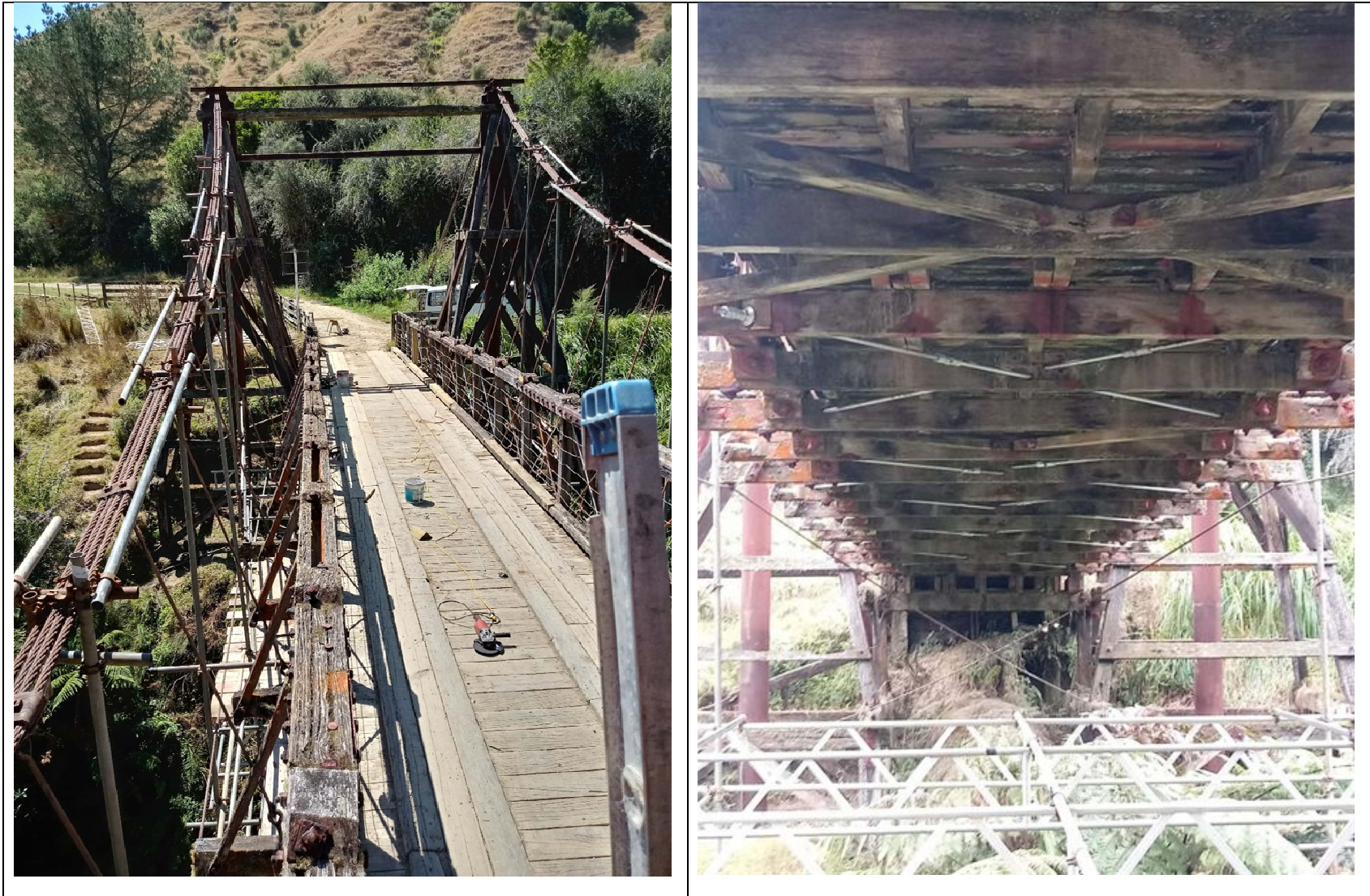
Figure 2: Kohuratahi Bridge Replacement Project
