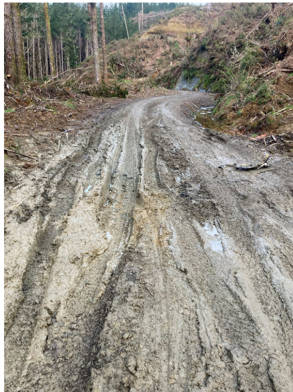
Figure 46 - Photo of Mangaoapa Road
