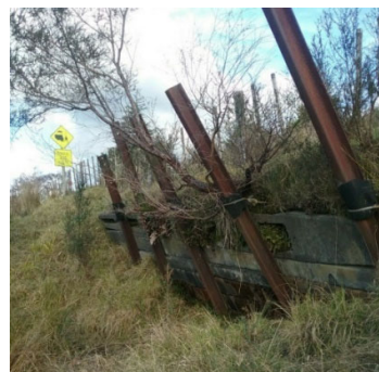
Wall #178: Mangaotuku Road
