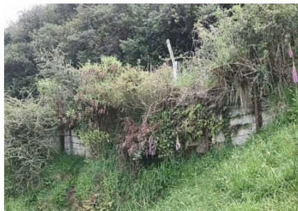
Wall number 227: Mangaehu Road
