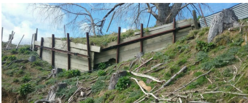
Wall #236: Mangaotuku Road
