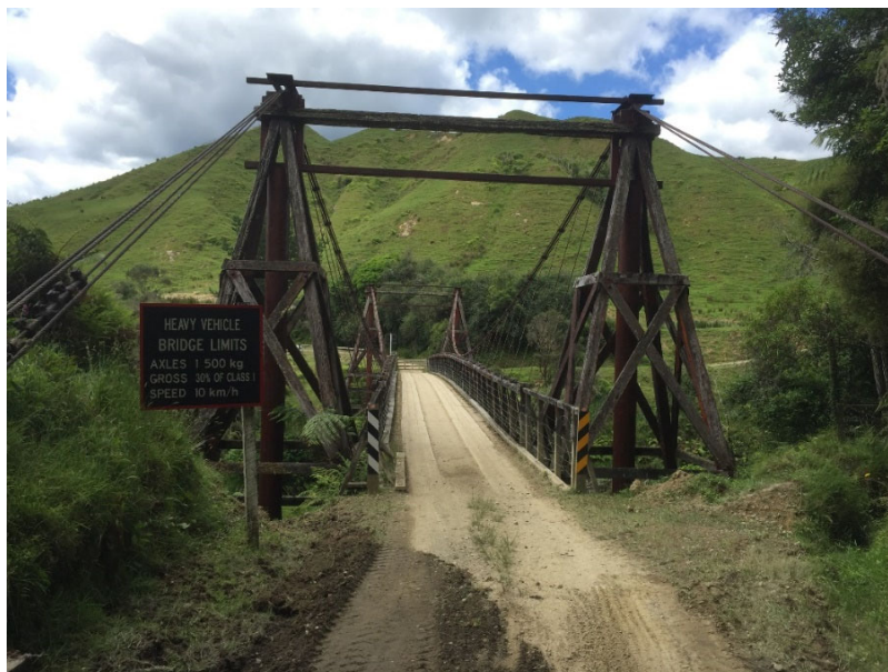
Figure 33 - Lower Kohuratahi Road Bridge
