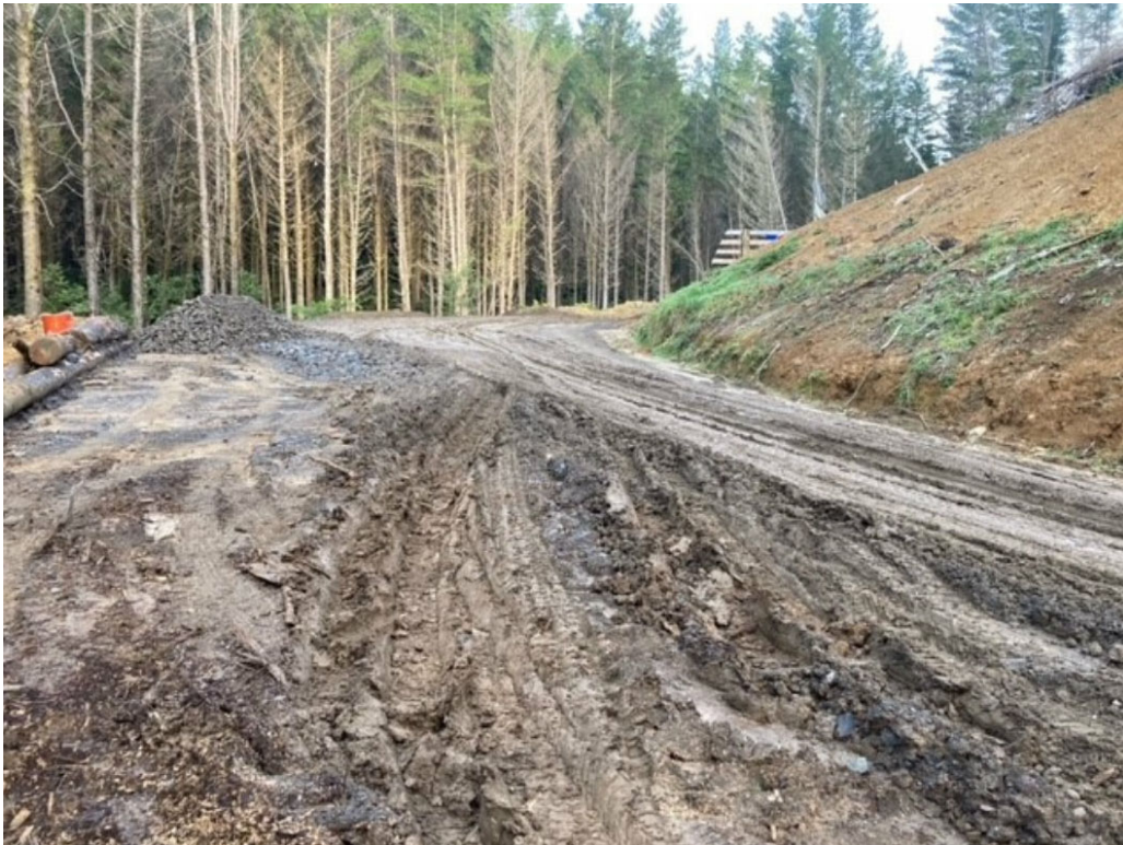
Figure 44 - Photo of Mangaoapa Road
