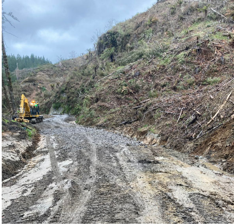
Figure 45 - Photo of Mangaoapa Road
