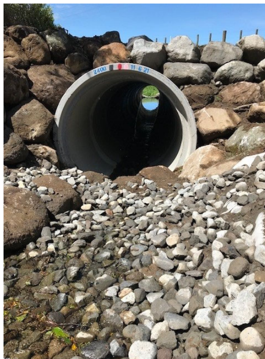
Newly installed culvert
