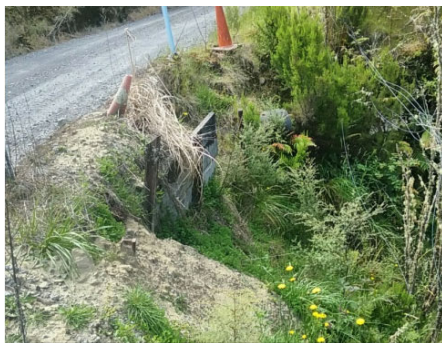
Wall #332: Mangaoapa Road
