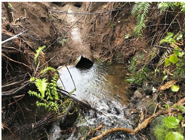
Existing culvert that was removed
