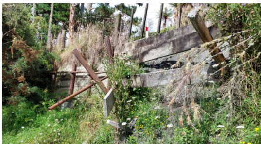
Wall #382: Mangaowata Road
