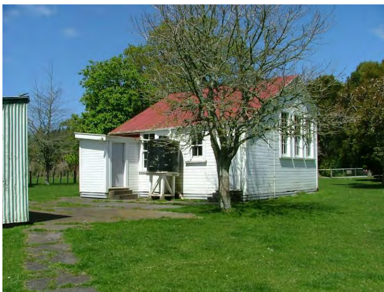
Te Popo Domain, former School Building
